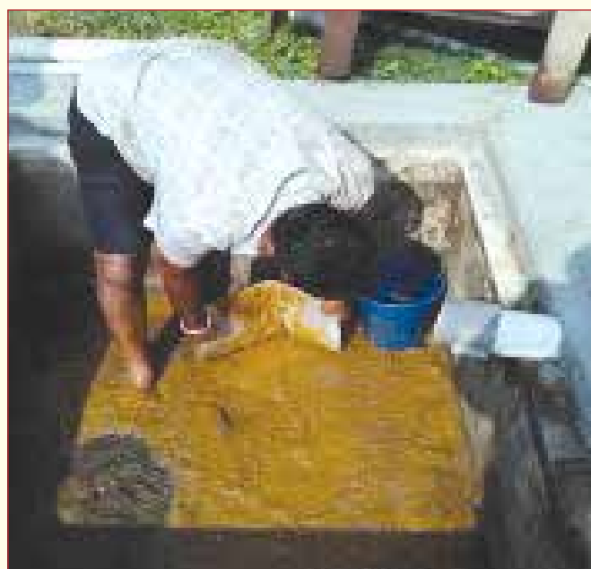
Fig 1. Removal of mucilage lodged on top of the sand-bed filtration pond
